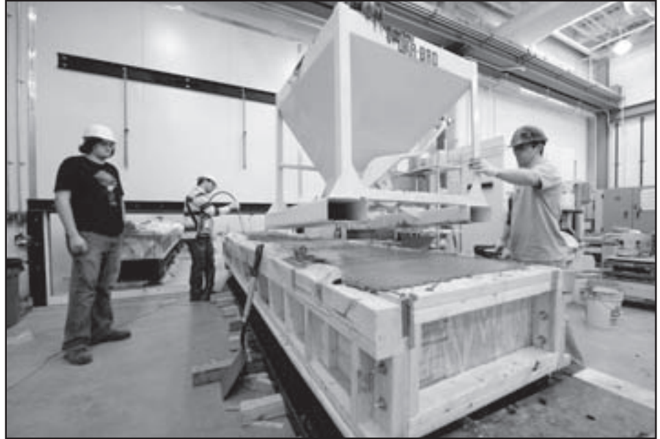
Purdue graduate students (from left) Paul Imbrock, Kambiz Raoufi and John Schlitter pour a test specimen of a new type of concrete for Indiana bridges that promises to reduce maintenance costs and allow bridge decks to last longer. Raoufi and Schlitter recently graduated. (Purdue University photo/Andy Hancock)
